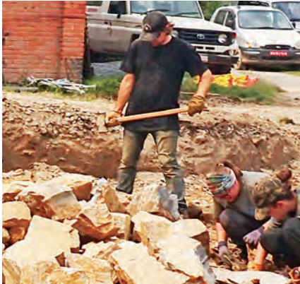
Breaking rocks for retaining wall
