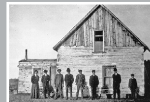
Renovated chicken house serving as the men's dormitory. Farm near Leduc, 1908
